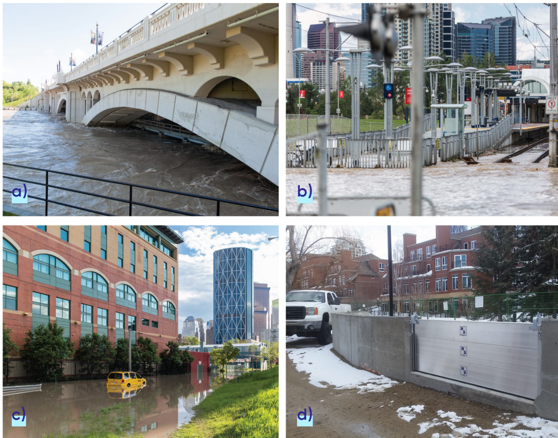
Figure 4.5: Damage and recovery from flooding in Calgary in June 2013: a) near record-high water levels on the Bow River, b) disrupted urban transportation, c) flooded City Centre, and d) West Eau Claire flood wall. Photos courtesy of: Shutterstock.
