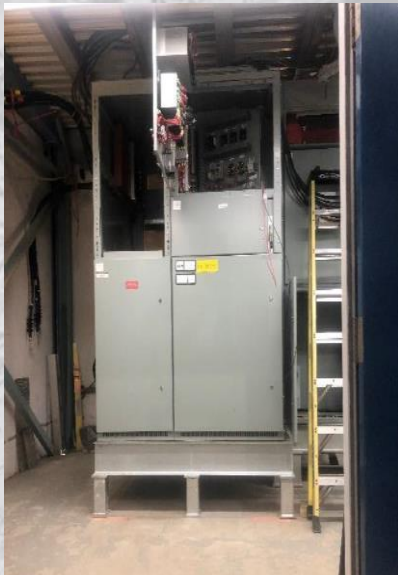
Above: Raising electrical equipment and floor in electrical room and raising floor in pump bay at Musquash Pumping Station.
