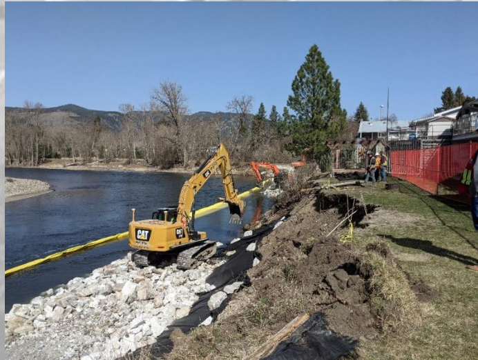
Below: Installation of revetment on the Kettle River to curb erosion after 2018 and 2020 freshets.
